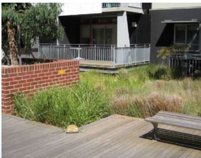
Figure 1: Stormwater diverted to and treated in the onsite bioretention system (wetland)
