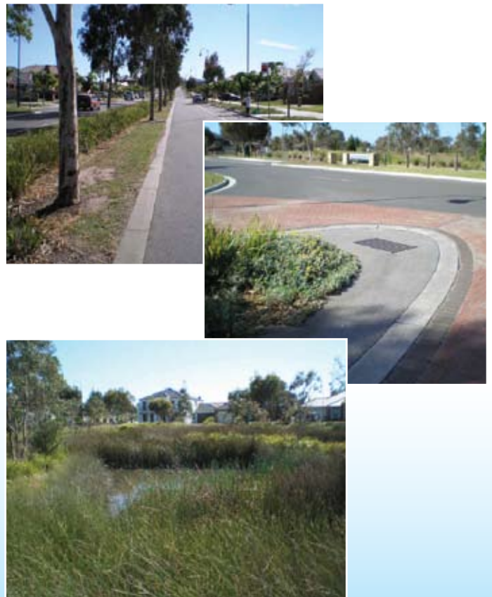
Figure 1: Main Boulevard, Flush kerbing, bioretention wetland at Lynbrook Estate
