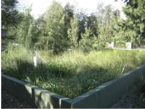
Monash Carpark Biofilter – October 2007
