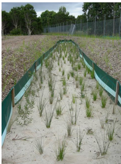
Second Ponds Creek Bioretention System
