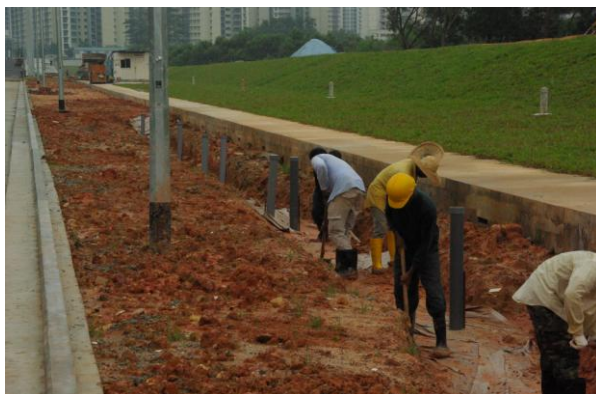
Biofilters under construction in Singapore
