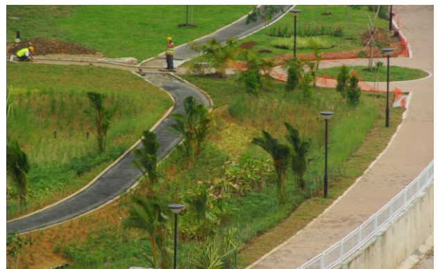
Biofilters under construction in Singapore
