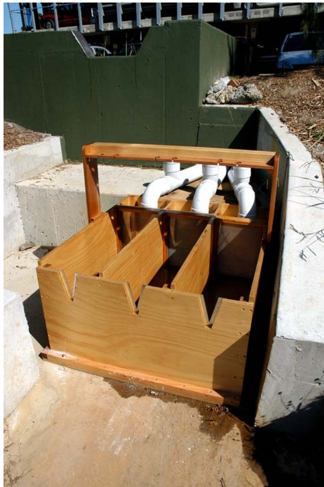
Figure S3.3 Downstream V-notch monitoring equipment, Monash Carpark Biofilter
