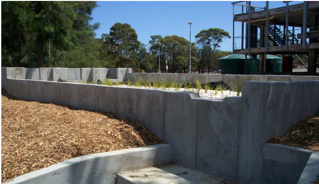
Figure S3.2 Monash University Carpark Biofilter facility
