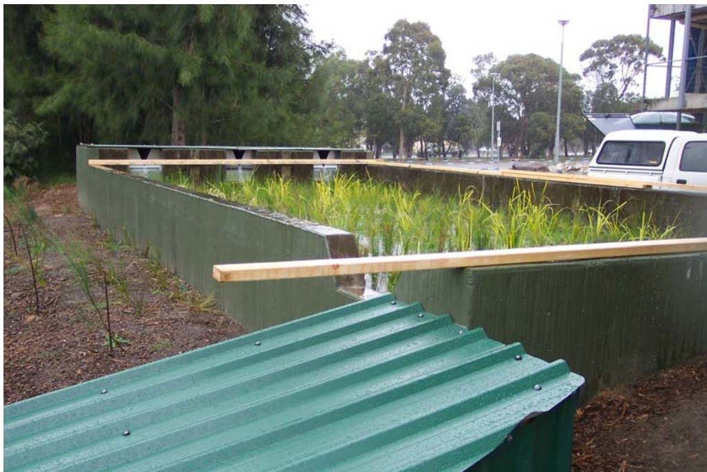
Figure S2.1 Downstream v-notch weir housing.
