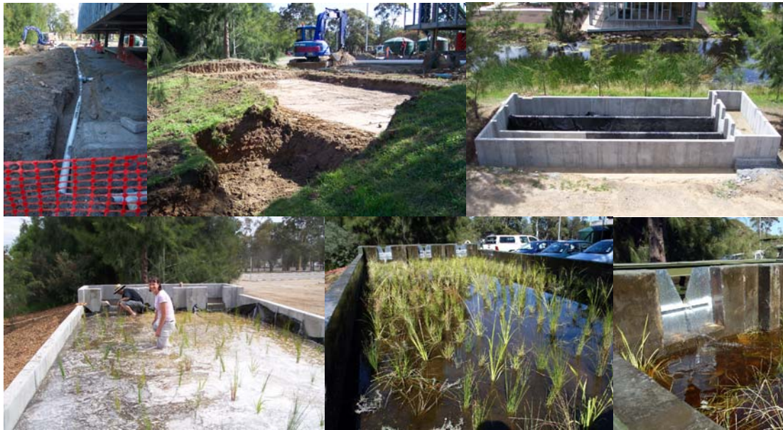
Construction of Monash University Car Park Biofilter
