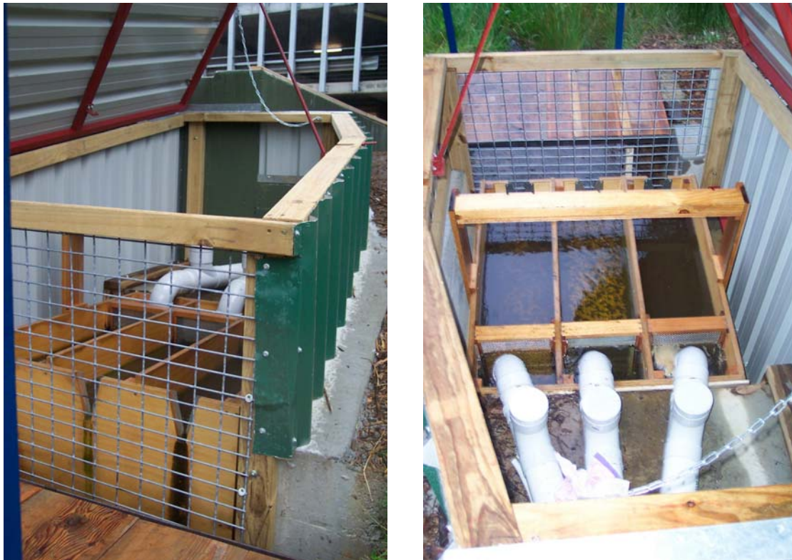
Figure S2.2 & S2.3 Downstream v-notch weirs.
