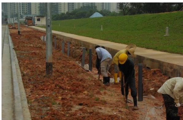
Biofilters under construction in Singapore
