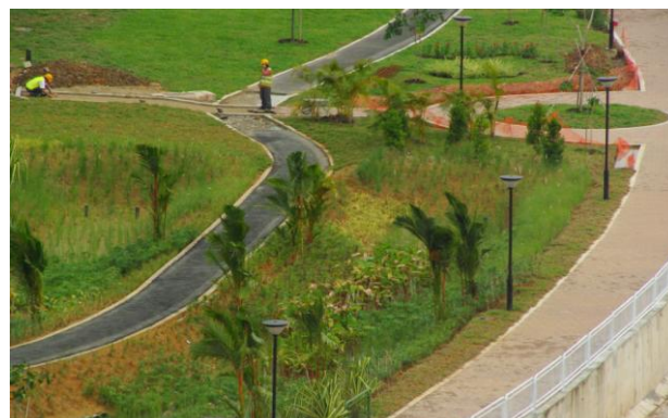
Biofilters under construction in Singapore
